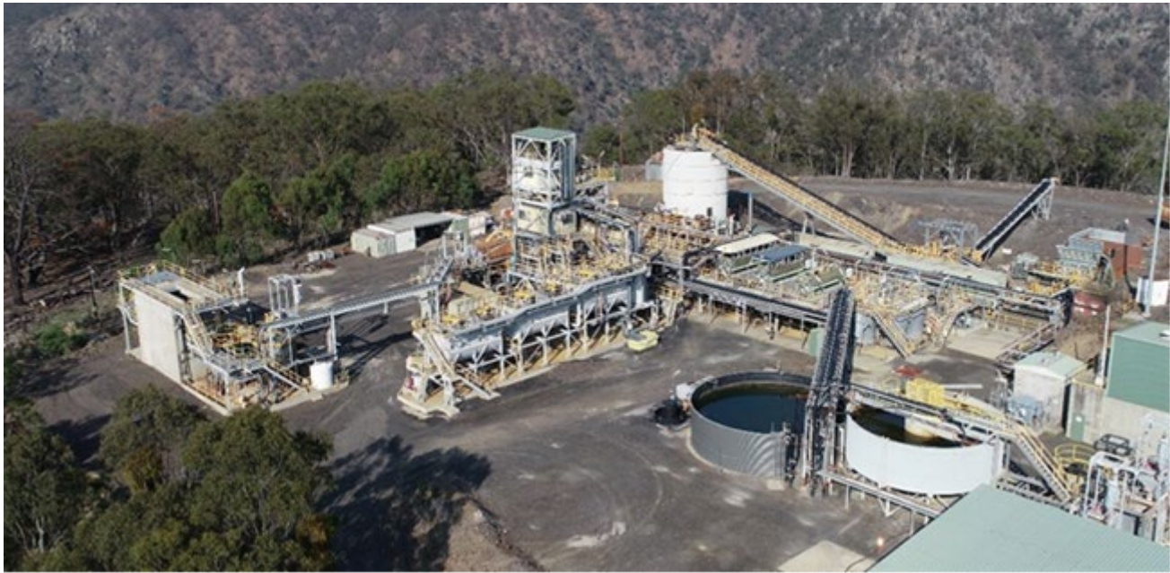
Figure 1. Hillgrove gold and antimony processing plant
