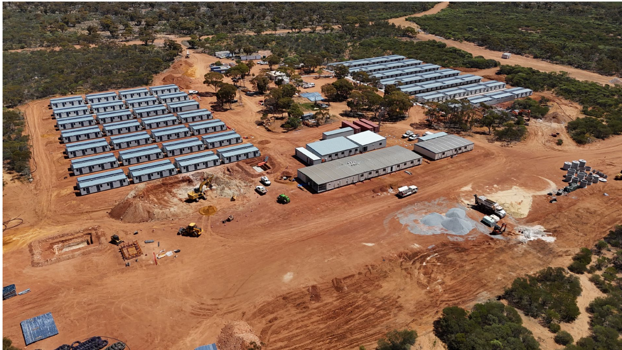
Mt Gibson Gold Project – accommodation village installation
