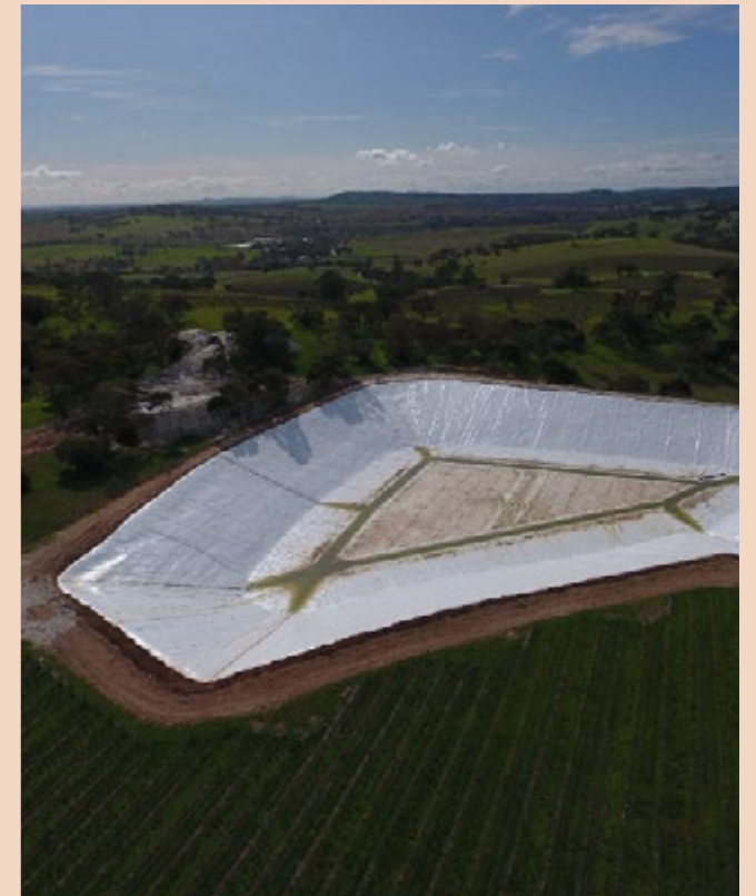
Dam cover replacement and cover installation at Zilm.
