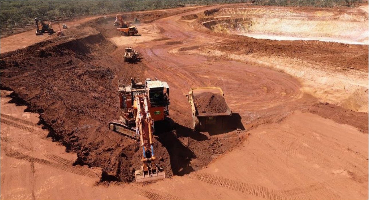
Figure 2: 200t excavator now on site and prioritising bulk waste movement in the Myhree open pit
