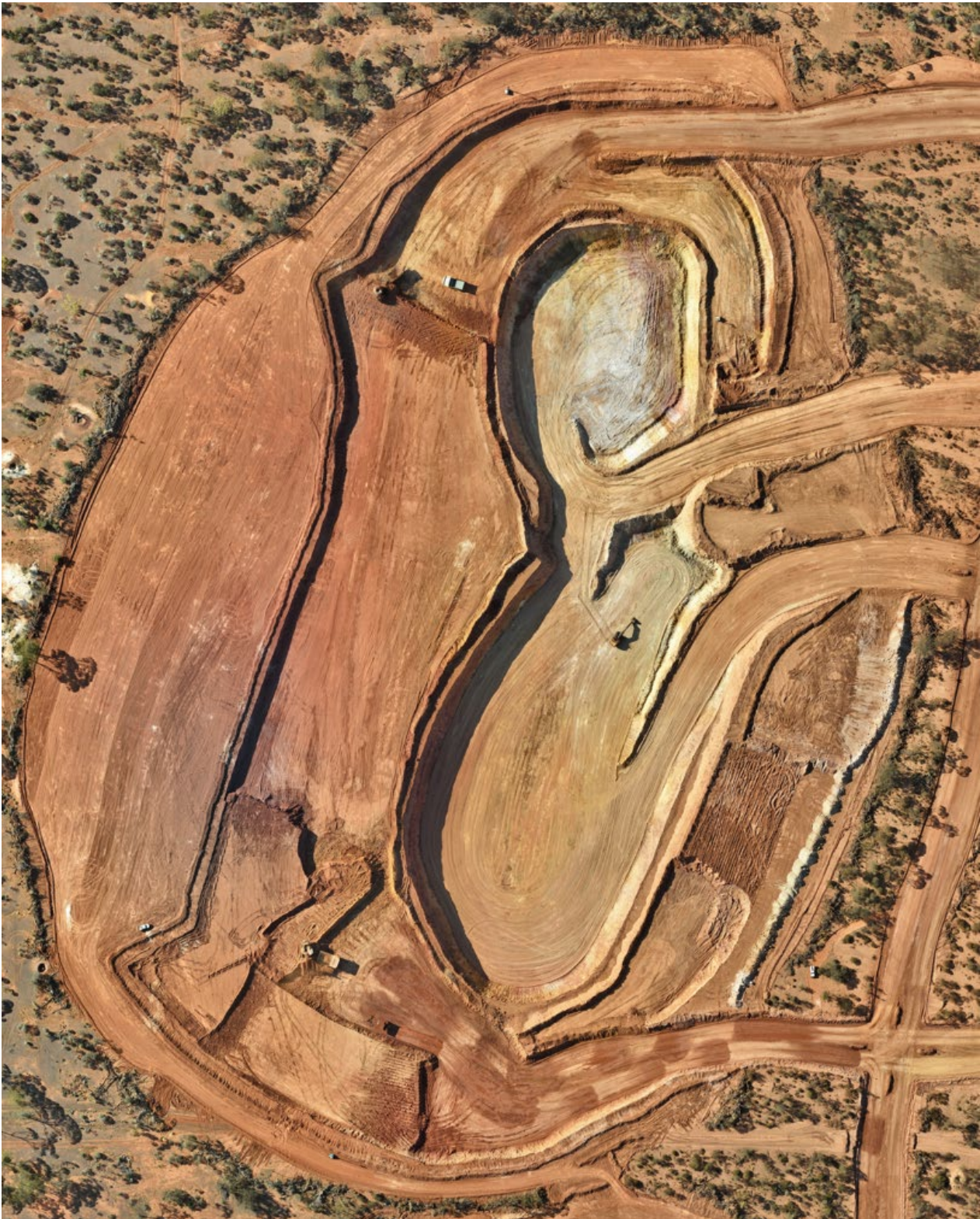
Figure 3: Aerial view of the Myhree open pit (north top of page)
