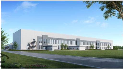
Precipitation & Filter Press plant
