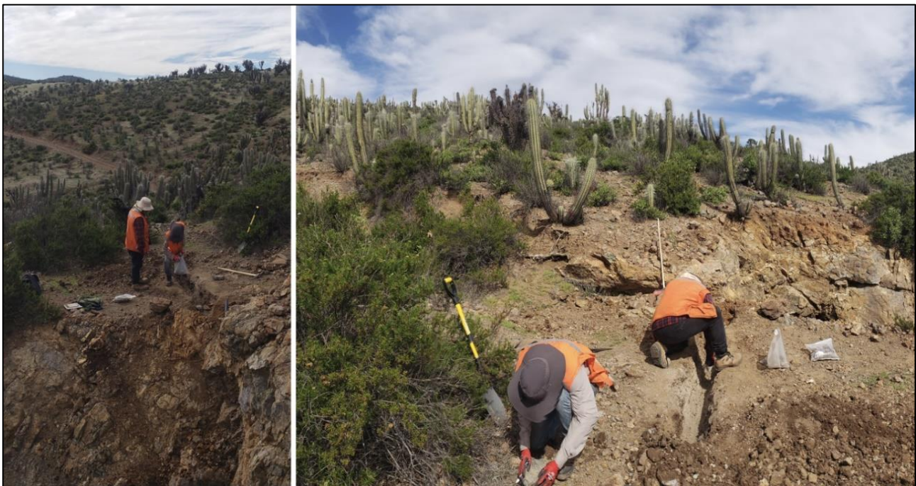
Figure 2: Trenching at an andesite outcrop with silica-albite-sericite alteration within a silicified and brecciated structure. Mineralisation shown to consist of quartz, iron oxides, and copper oxides. Samples CPO0009117- CPO0009118- CPO0009119 Trench 1 (5.5m at 0.88% CuEq).
