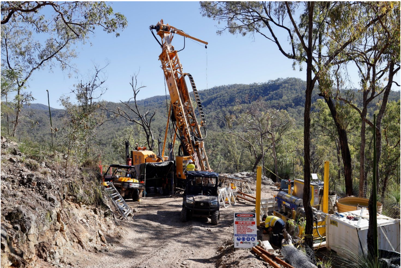
Figure 12. Drill rig in action, Briggs Central
