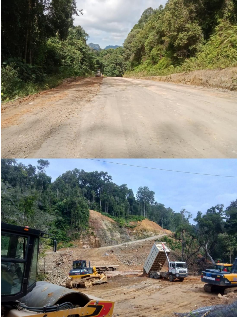
Road & Bridge Construction from Pit 3 to KM52
