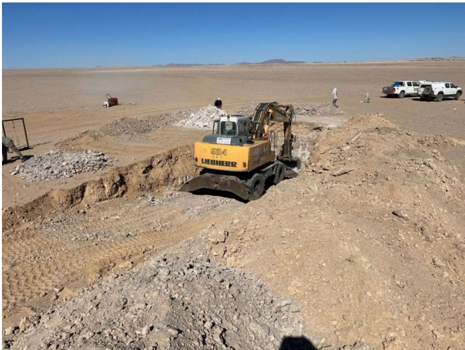
Figure 5 – Test Pit Excavation at Koppies Resource
