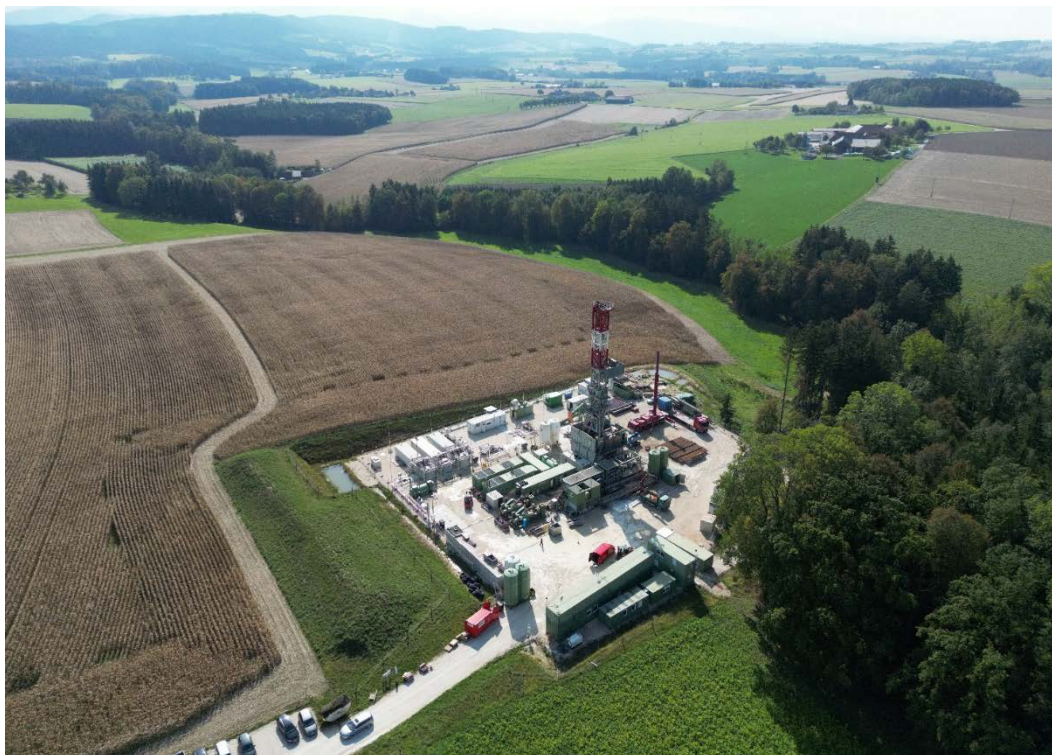
Figure 2: The RED E-202 rig on location at the LICHT-1 well site
