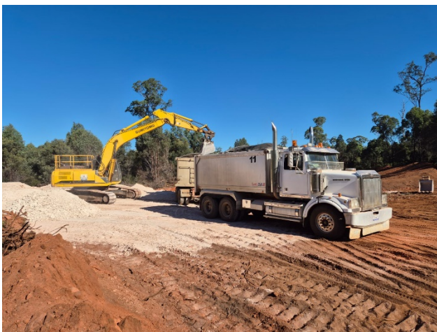
(above) test pit at the Toondoon Kaolin Project
