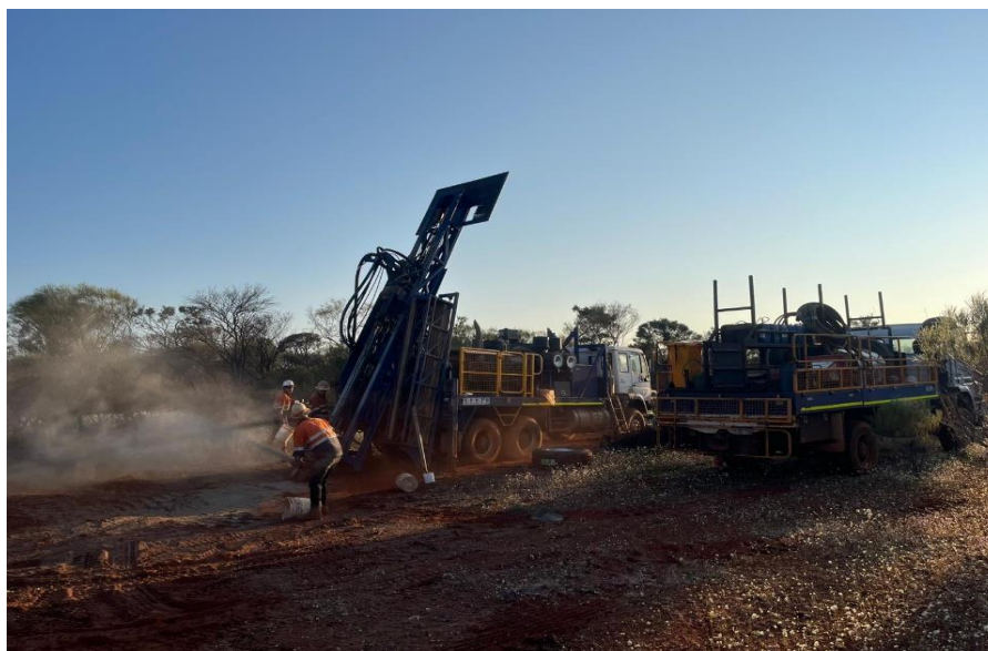
Picture 1: Ragland AC rig on site at Wildflower - First Hole this morning "The Hunt has Begun".
