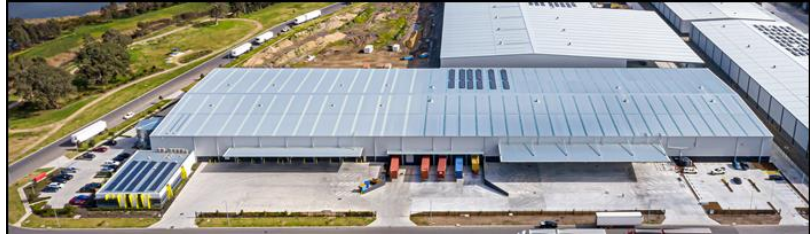
NTAW Distribution Centre in Melbourne
