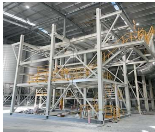
Structure ready for installation of Classifiers
