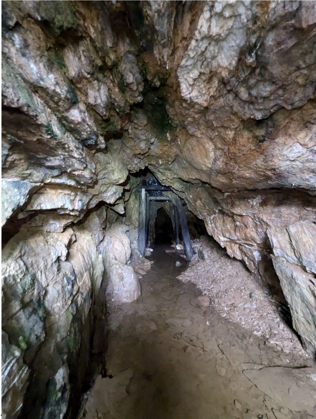
Figure 7: Inside entrance to Old Antimony mine adit 1
