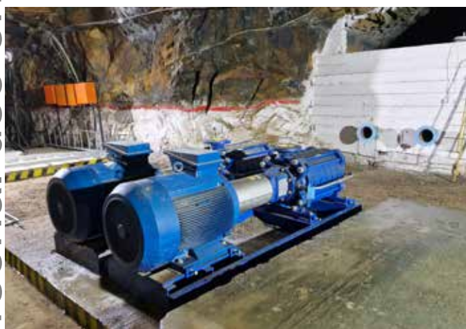
Photo 3: Underground 178m Level Multi-Stage Pumps.
