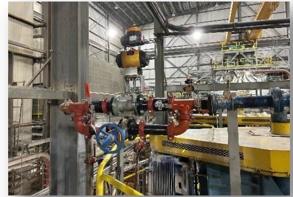
Picture 3: New air distribution valves and flowmeters
