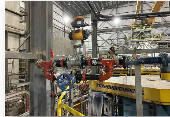
Picture 3: New air distribution valves and flowmeters
