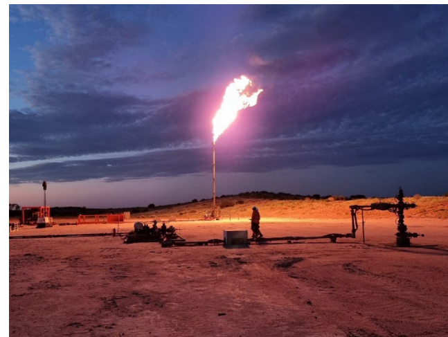
Gas flare from Kiwi-1 wellsite at 1.7 mmcf
