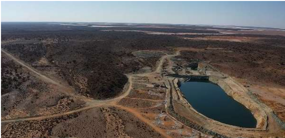
Figure 4: Devon Open Pit, oblique view looking along strike to the northeast
