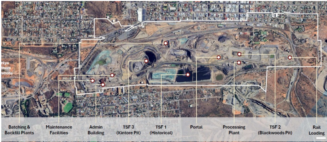
Plan view of the Rasp Mine Mining Lease and outline of surface infrastructure.
