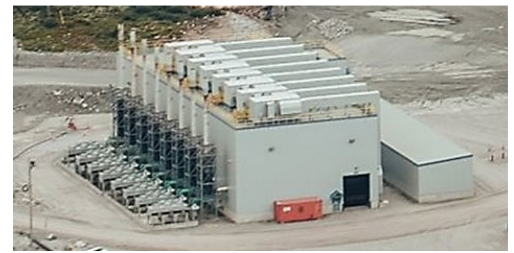
Figure 6. LNG-fired power station with a total capacity of 16MW
