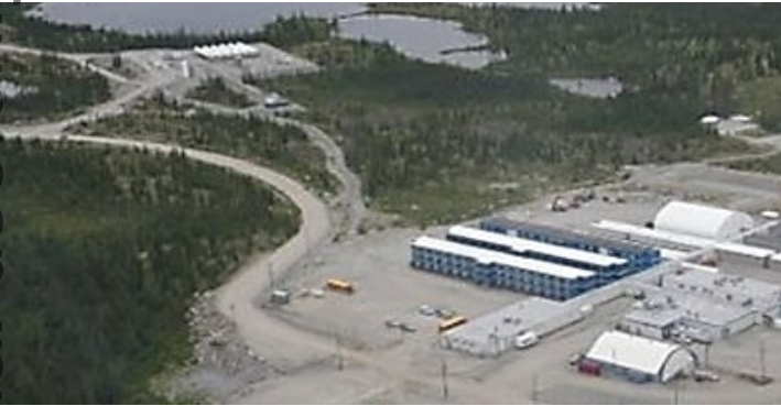
Figure 1. Access Road and Accommodation Camp (capacity for 330 pax)
