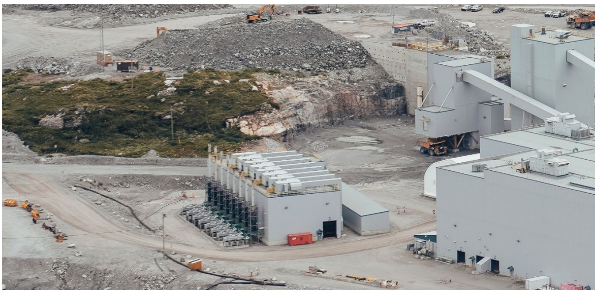
Figure S20: Natural Gas Power Plant – Renard
