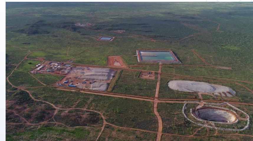
Aerial photo of existing infrastructure at Browns Range
