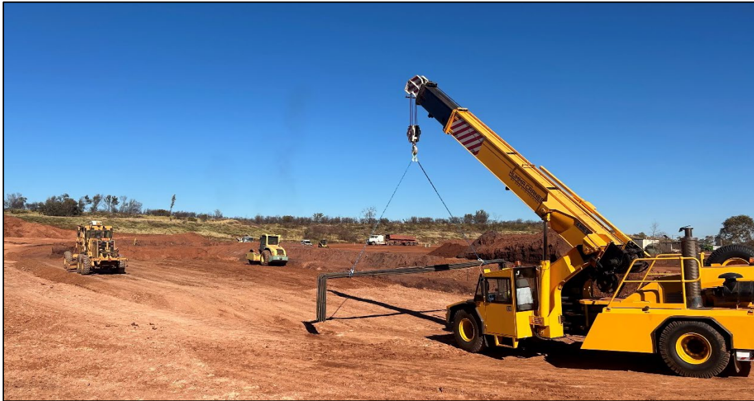
Photo 1: Commencement of Construction of Nobles CIL Gold Processing Facility – June 2024
