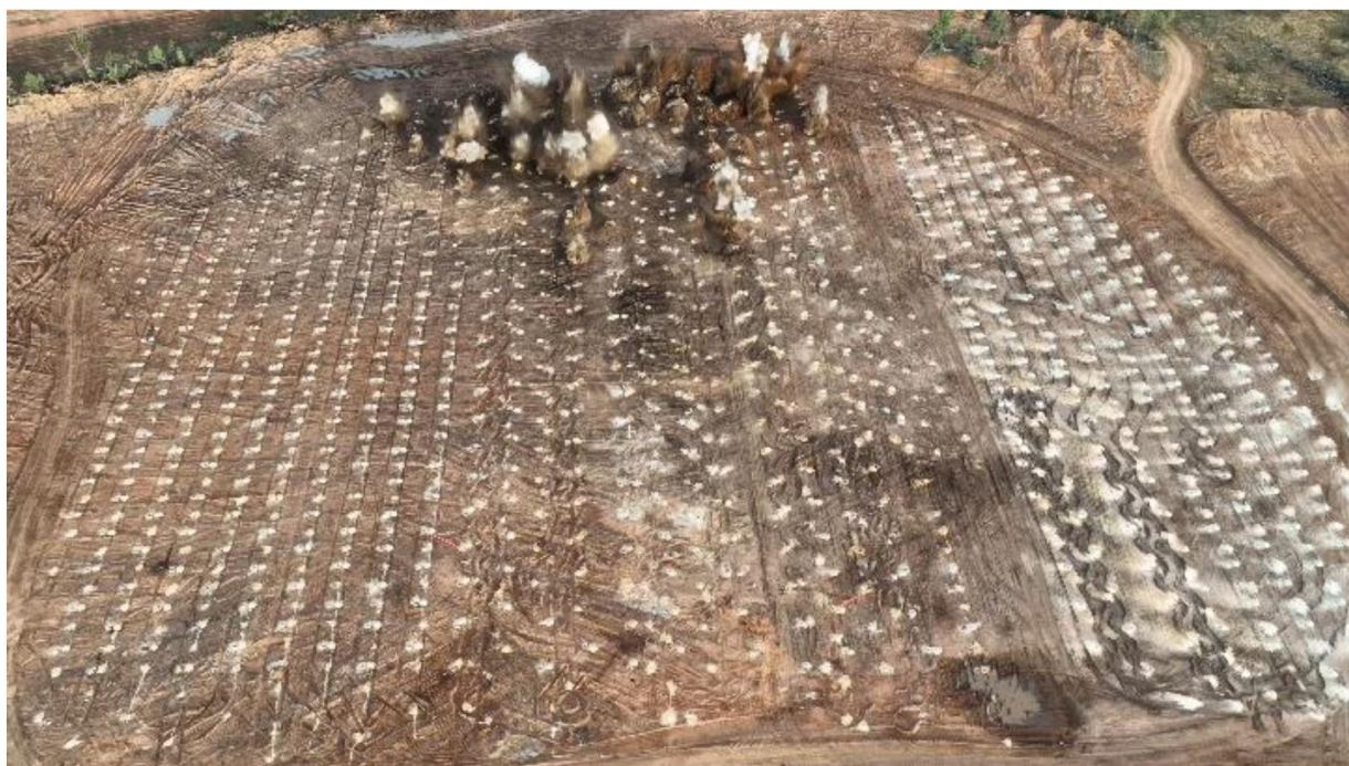
Figure 1: Open pit blast.
