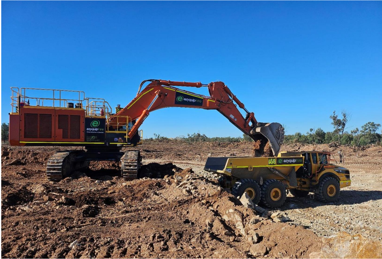
Figure 2: Open pit excavation haulage
