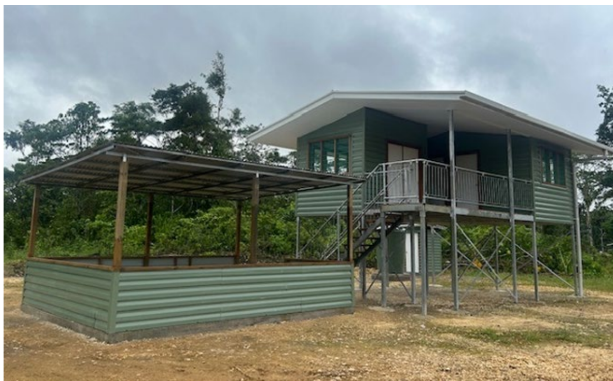
Relocation house completed during the reporting period
