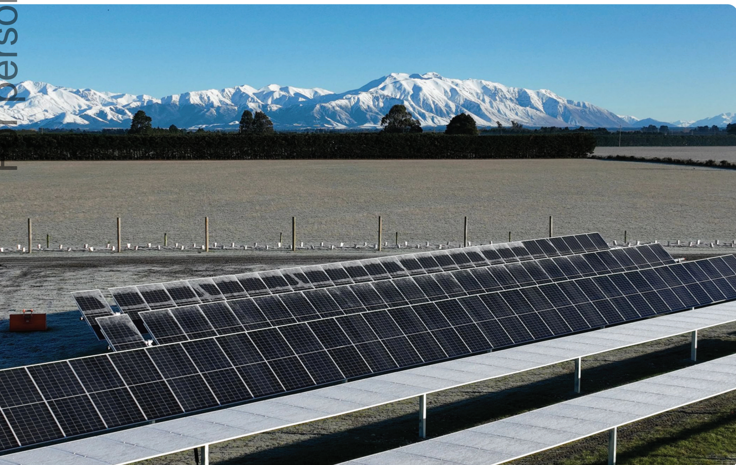
Lauriston Solar Farm - under construction
