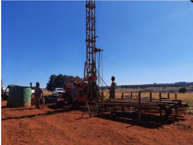
Figure 2: Diamond drill rig is in operation in CODA North
