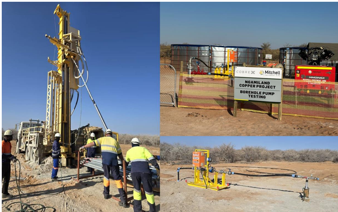
Figure 3. Drilling and development of pumping well PW02.
