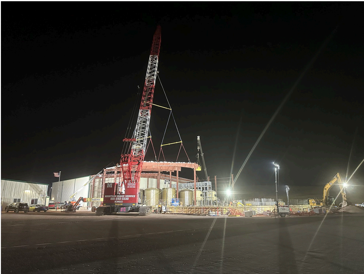
Figure 1: Nighttime placement of roofing structure
