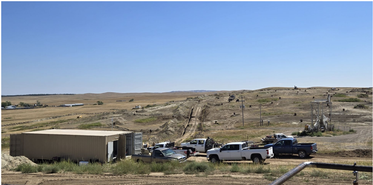
Figure 6: MU-3, HH-11 building in the foreground with installed wells in background
