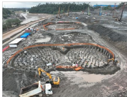
Liquid storage tanks
