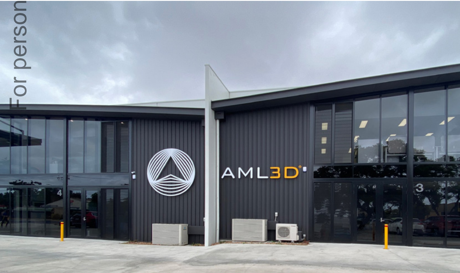
AML3D's Adelaide Technology Facility.
