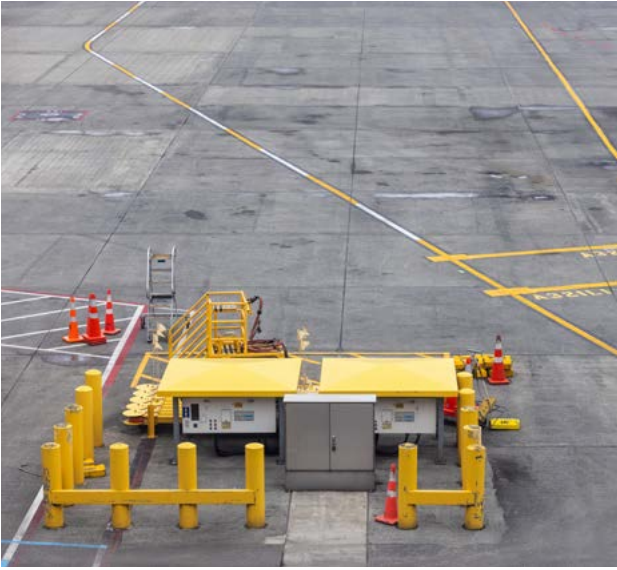
Ground power units enabling international aircraft to connect to NZ's low-carbon electricity supply.
