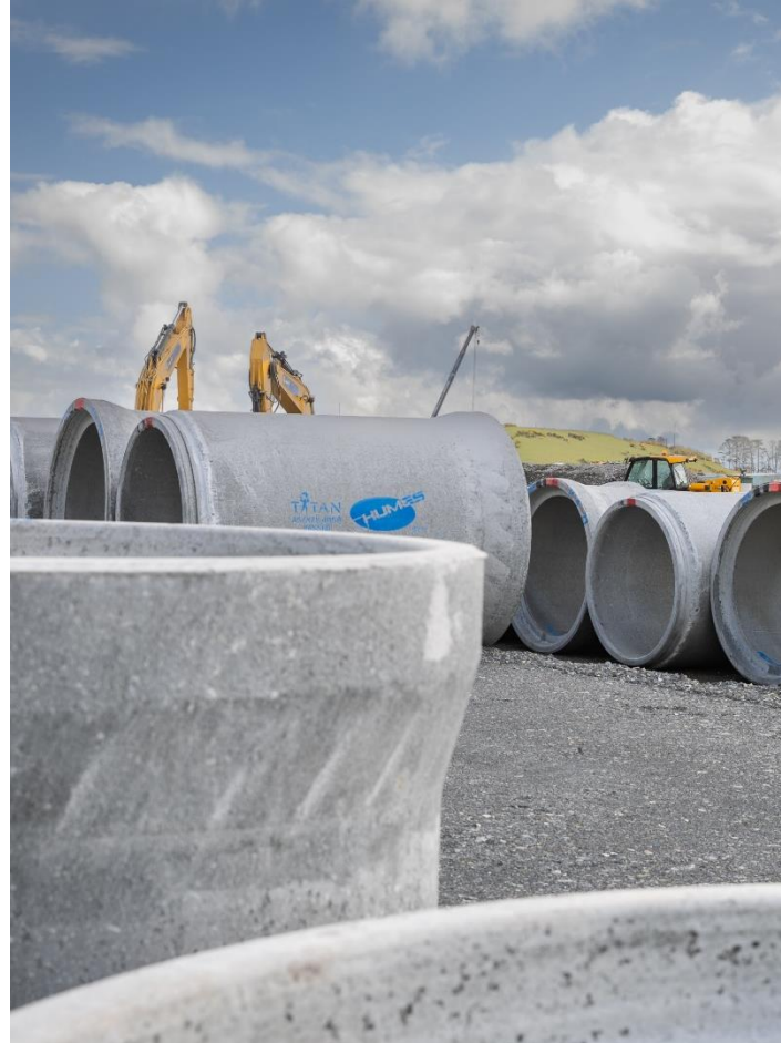
Stormwater pipes awaiting installation
