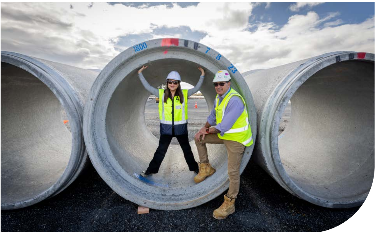
7 Pre-implementation Programme Manager Adrienne Khor and Mark Blanchard, Construction Operations Manager, demonstrate the size of stormwater pipes installed as part of a 3.5km network.
