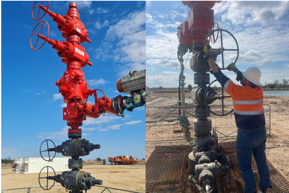
Servicing of well head at Daydream-2
