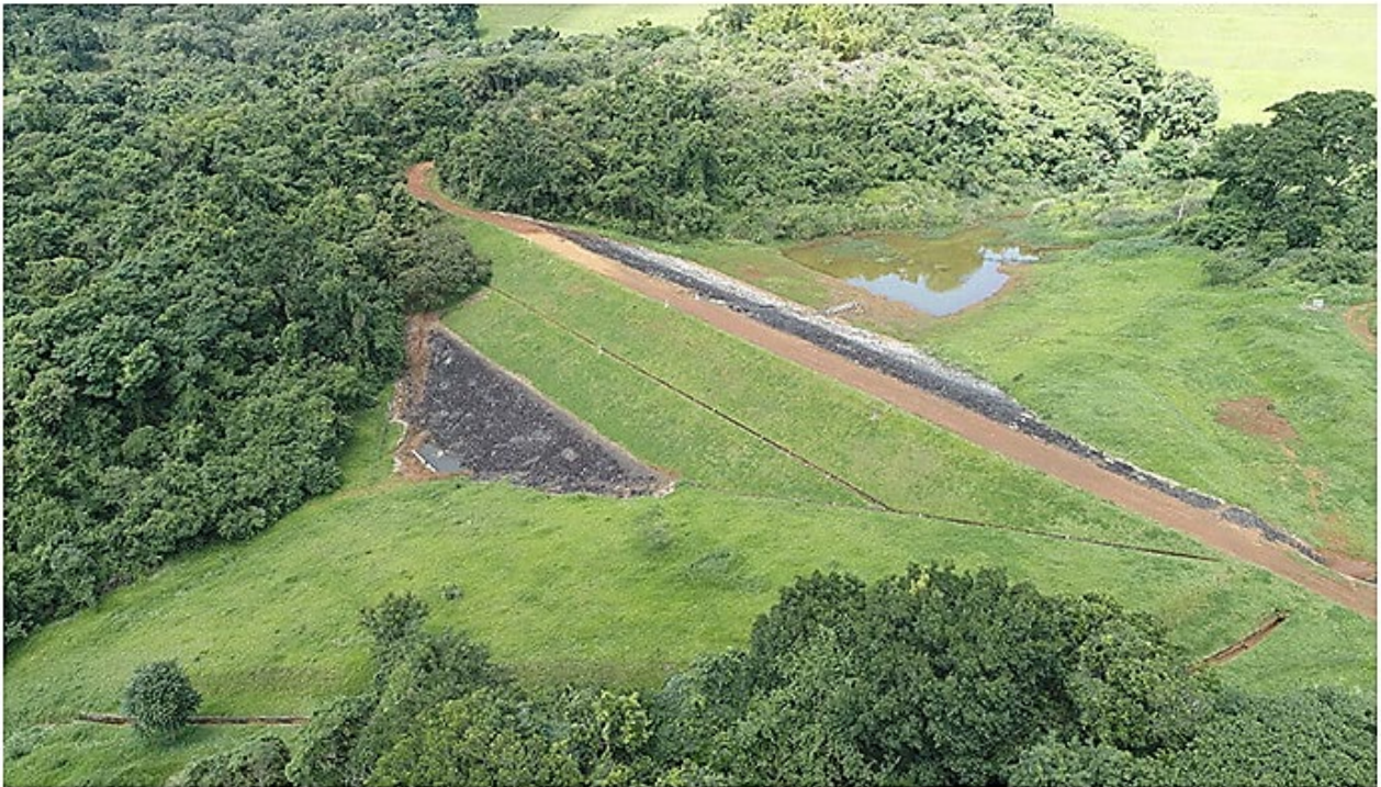
Figure 2 – photo of Dam D. Source: https://cbmm.com/en/our-company/our-dams
