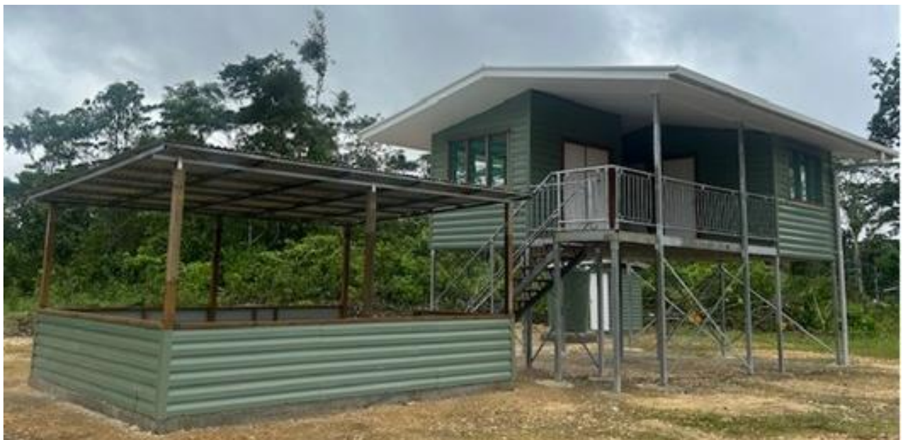
Figure 8: Example of completed community house
