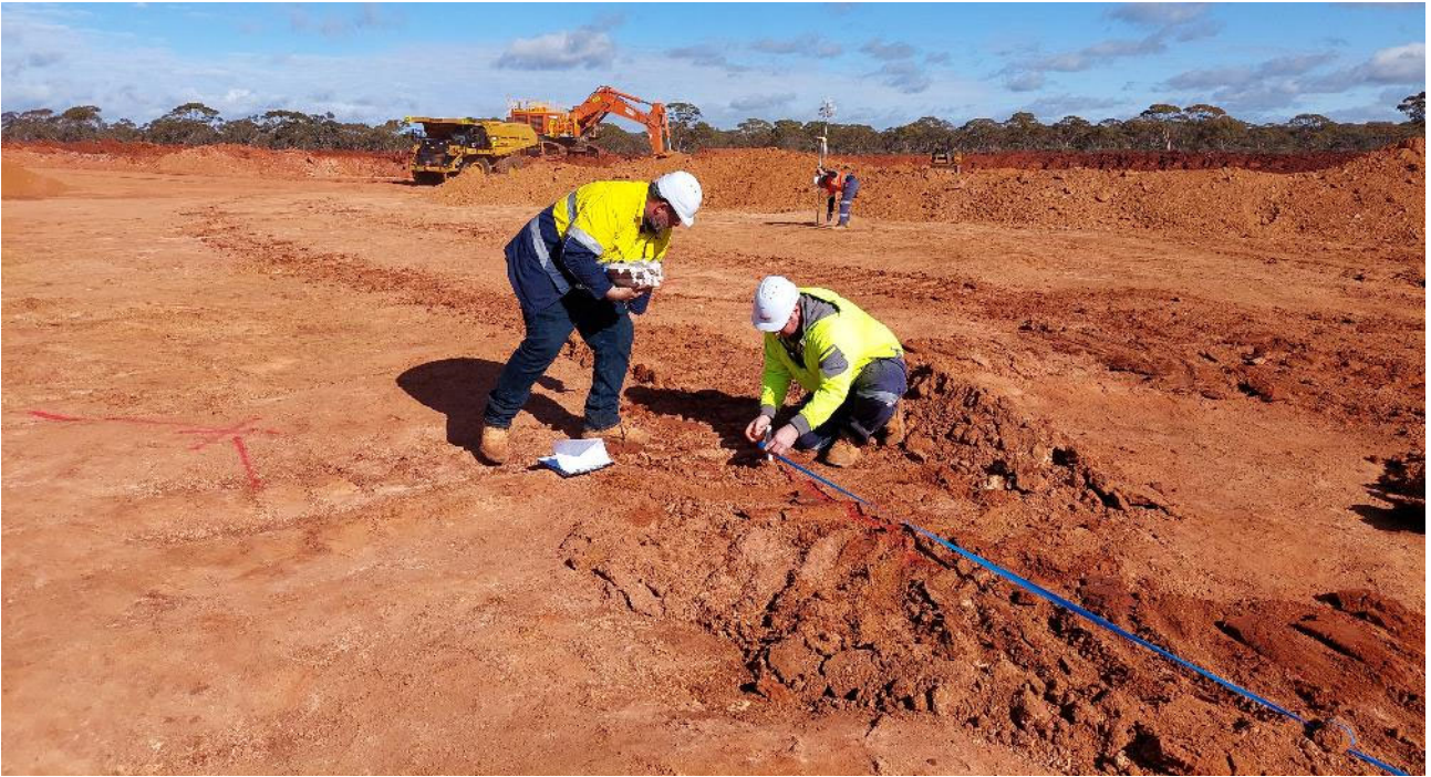
Figure 2: First Ore being marked up at the Myhree open pit (pink >3.0g/t Au, blue <3.0g/t Au).
