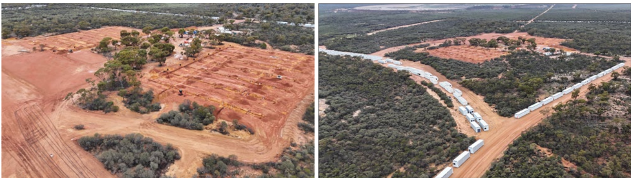
Mt Gibson Gold Project – accommodation village installation
