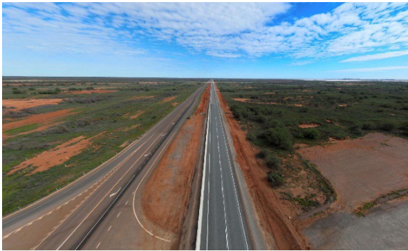
Sealing of dedicated haul road is progressing
