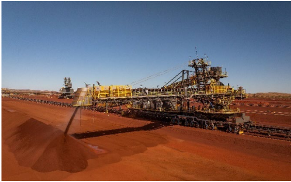
Stacker in operation at Ken's Bore
