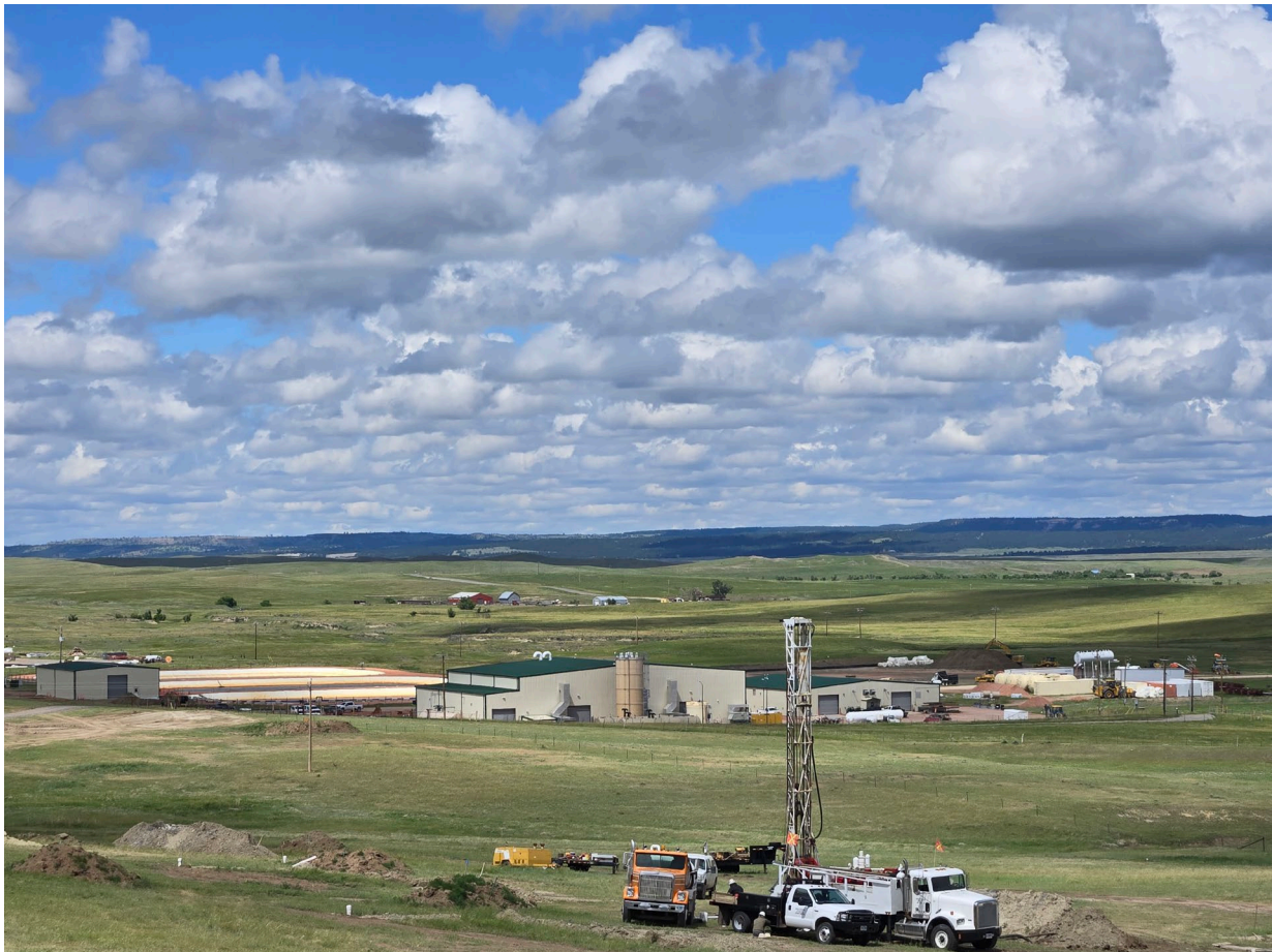
Figure 4: Active well installation at Mine Unit 3. Ross Plant in background
