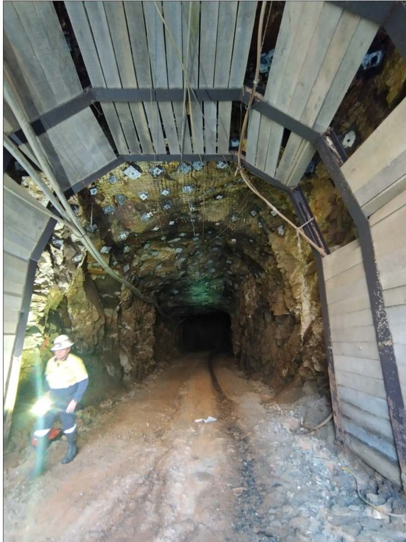
Picture – Photograph from Bullen portal and decline development June 2024
