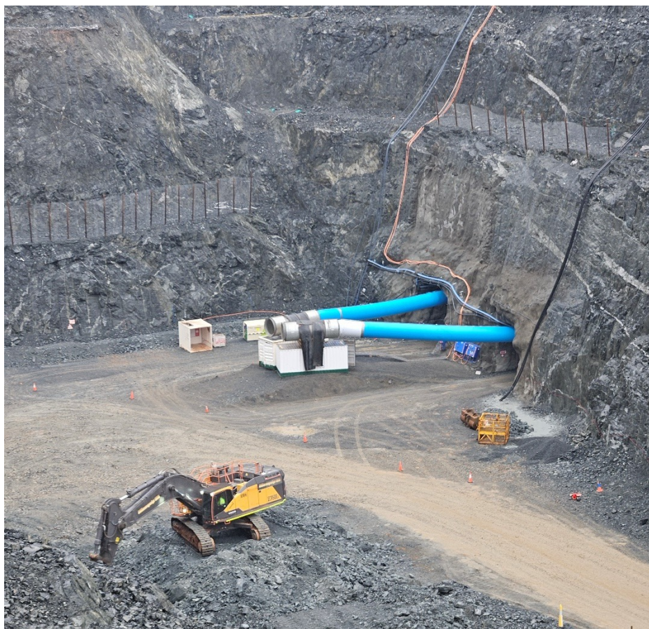
Picture – Scotia portal and ventilation drive progressing ahead of plan.
