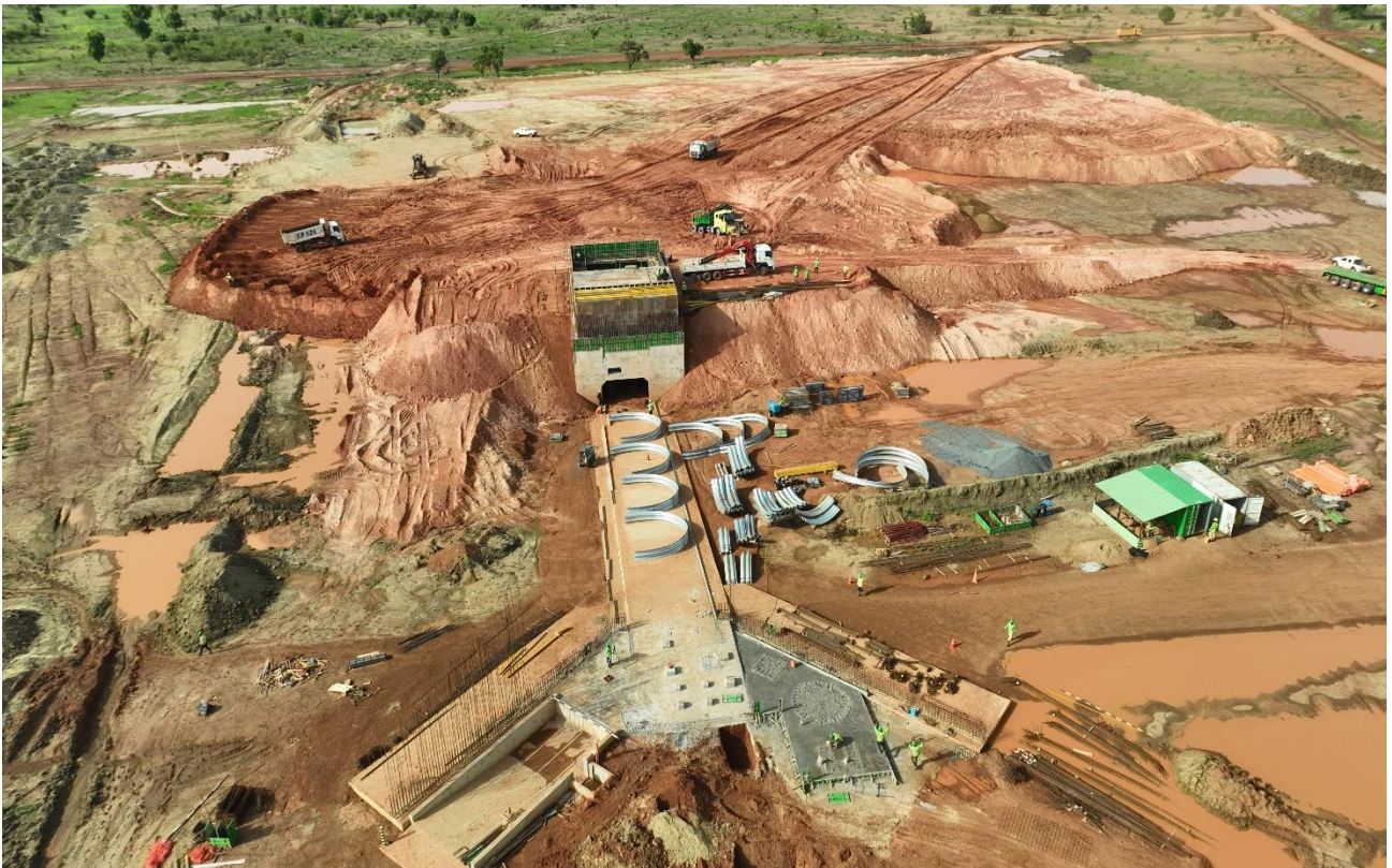
Kiaka Primary Crusher Area
