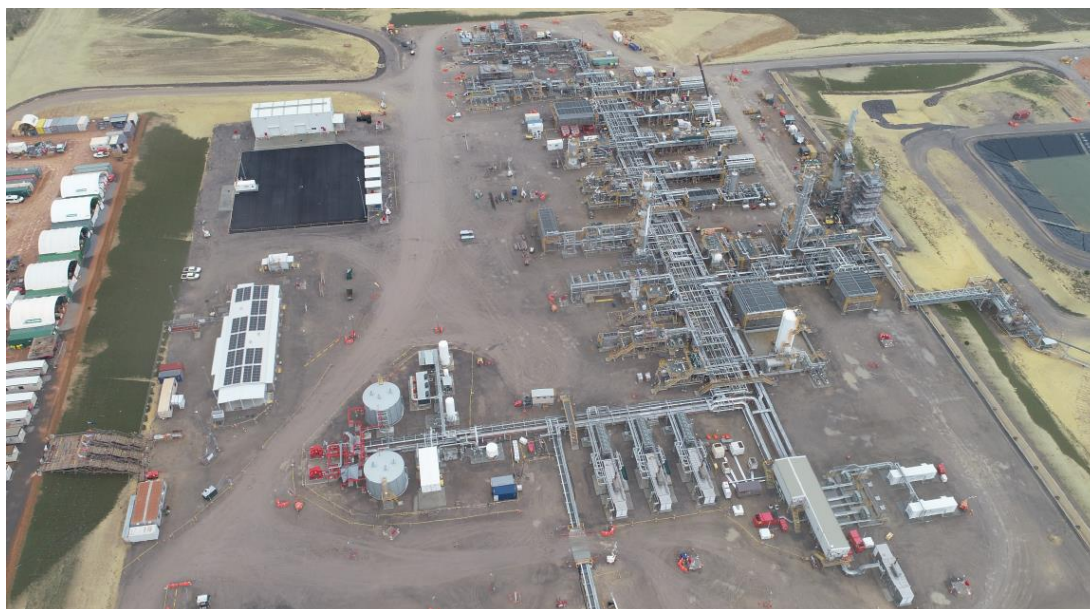
Waitsia Gas Plant during pre-commissioning
