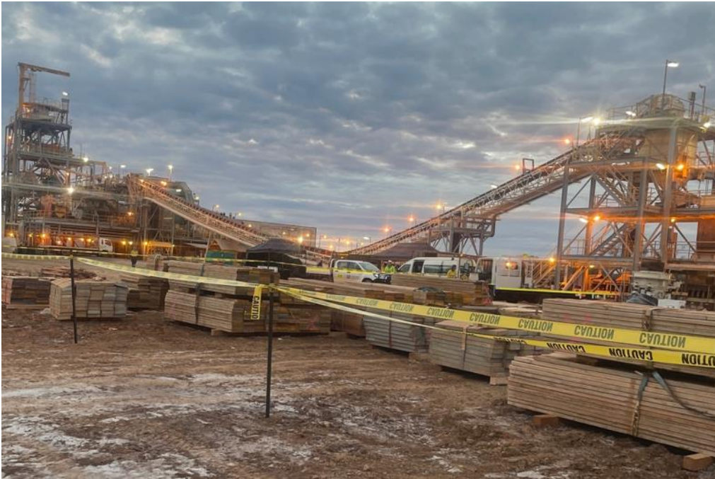
Figure 6. Laverton mill re-start - Scaffolding delivered
