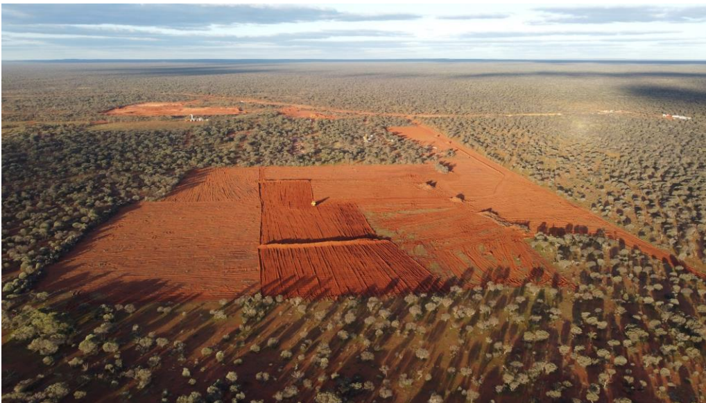
Figure 7. Hub open pit - Clearing site
