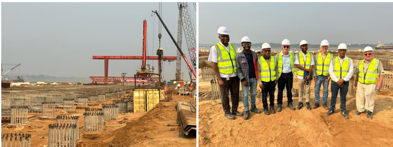
Figure 1. Visiting Porto do Caio Stage 1 Quay which is scheduled for completion in December 2025.
