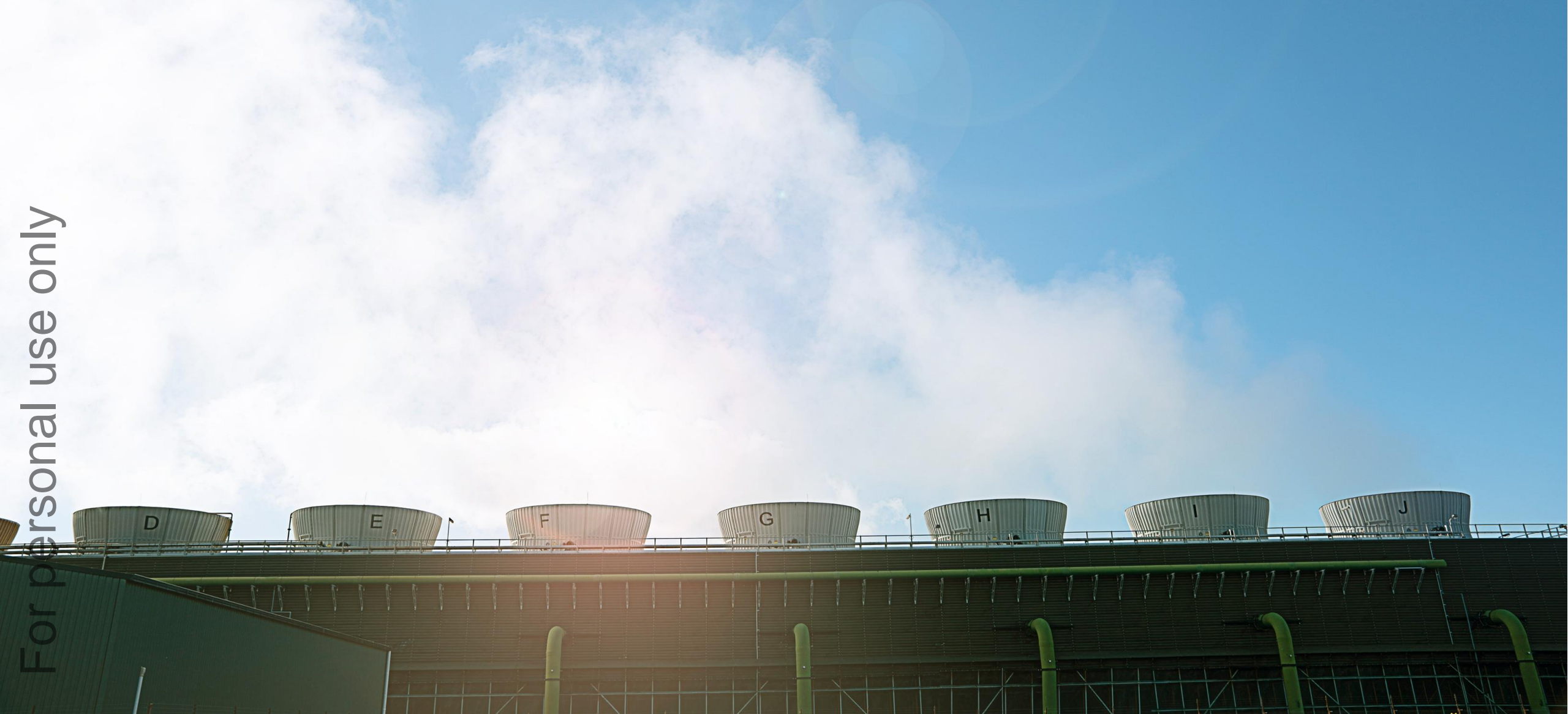
Ngā Awa Pūrua cooling tower
