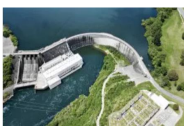
Karāpiro (1946) 101MW 515GWh
