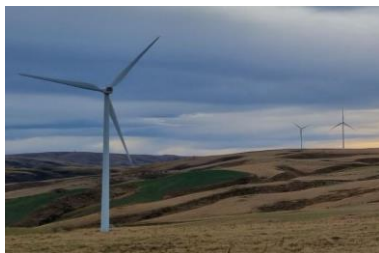
Mahinerangi (2011) 36MW 100GWh
