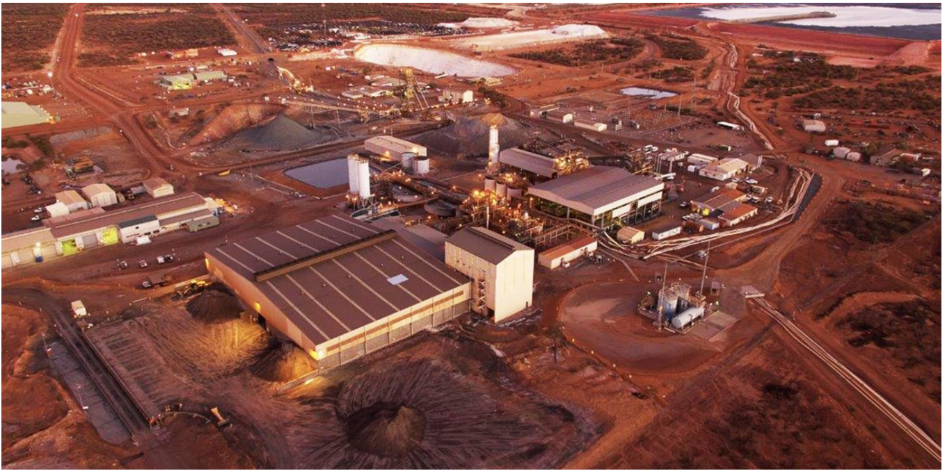
Figure 1: Processing plant at Golden Grove Mine, WA
