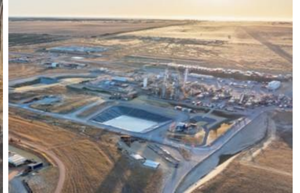
Waitsia Gas Plant
