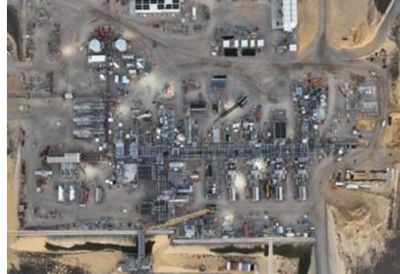
Waitsia Gas Plant
