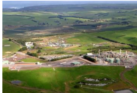
Otway Gas Plant
