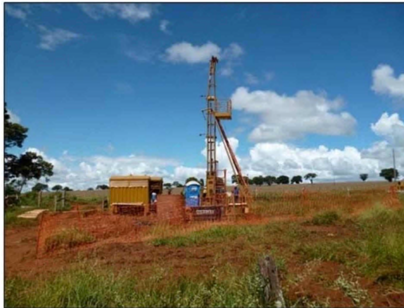
Figure 6-5 – Drilling equipment in operation in borehole PMC-FD-0074
